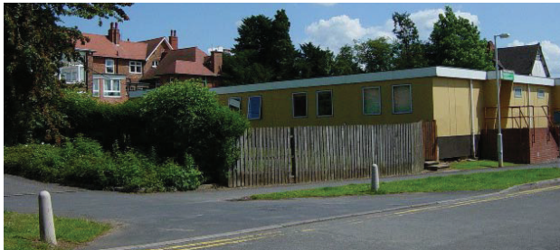
View of existing Health Centre
